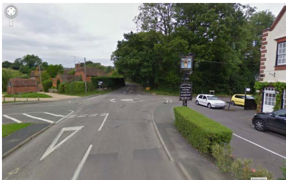
Shere Road (B2127 Ockley Road jnc) looking north
